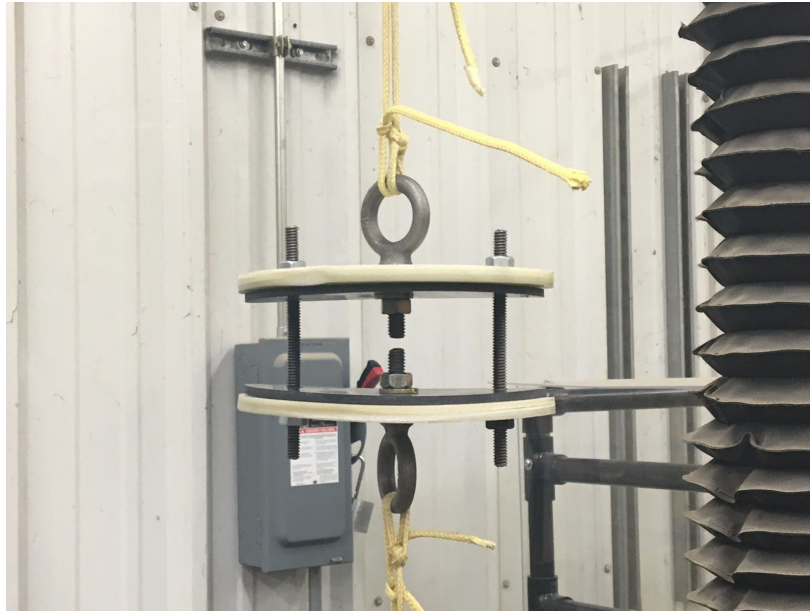
Figure 3.8.7. Deformation of fiberglass bulkheads
